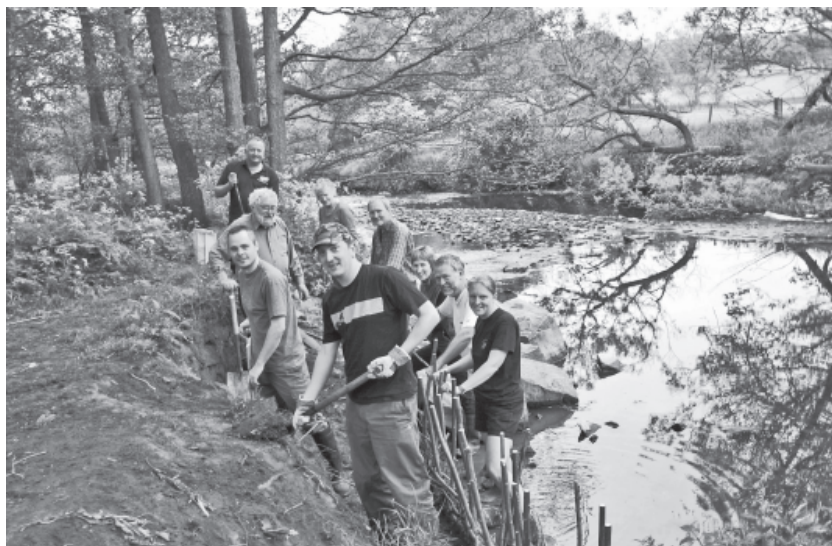
Lanchester Valley Conservation Group, with Durham County Council Ranger Service, weave willow strips to contain the river bank at Malton, on Sunday June 6th.
