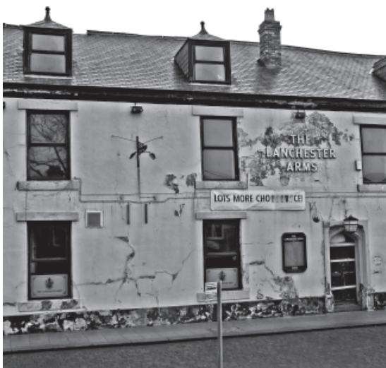
The sorry state of the Lanchester Arms. Note the missing ridge tile.
