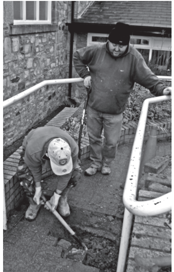
Bill and Paul of Poplar Builders prepare the trench to relay the gas pipe
