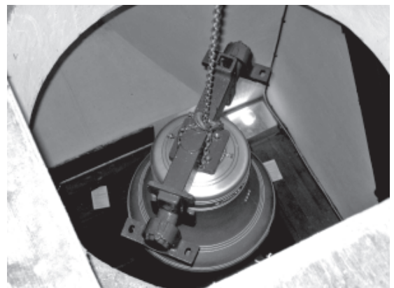
View of one of the bells on the final phase of its journey into the belfry
