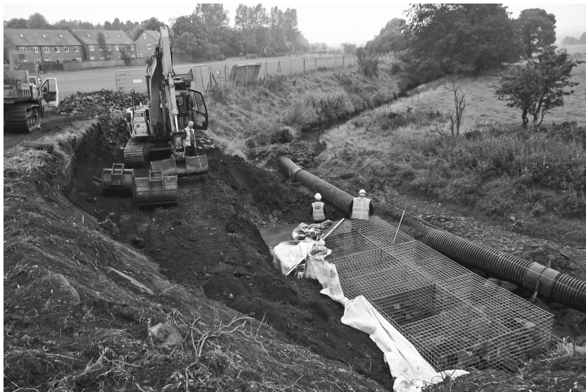
The work being undertaken to stop erosion on the banks of Smallhope Burn.
