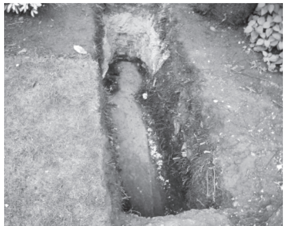
The view of the culvert underneath the first tree to be removed, showing the roots of the trees.
