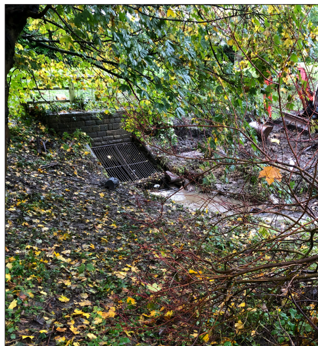
Above: This shows the culvert after it had been cleaned out – the grid clearly visible and water level much reduced.
